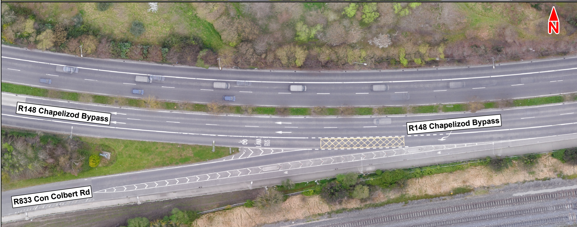
B) R148 CHAPELIZOD ROAD/R833 CON COLBERT ROAD JUNCTION
