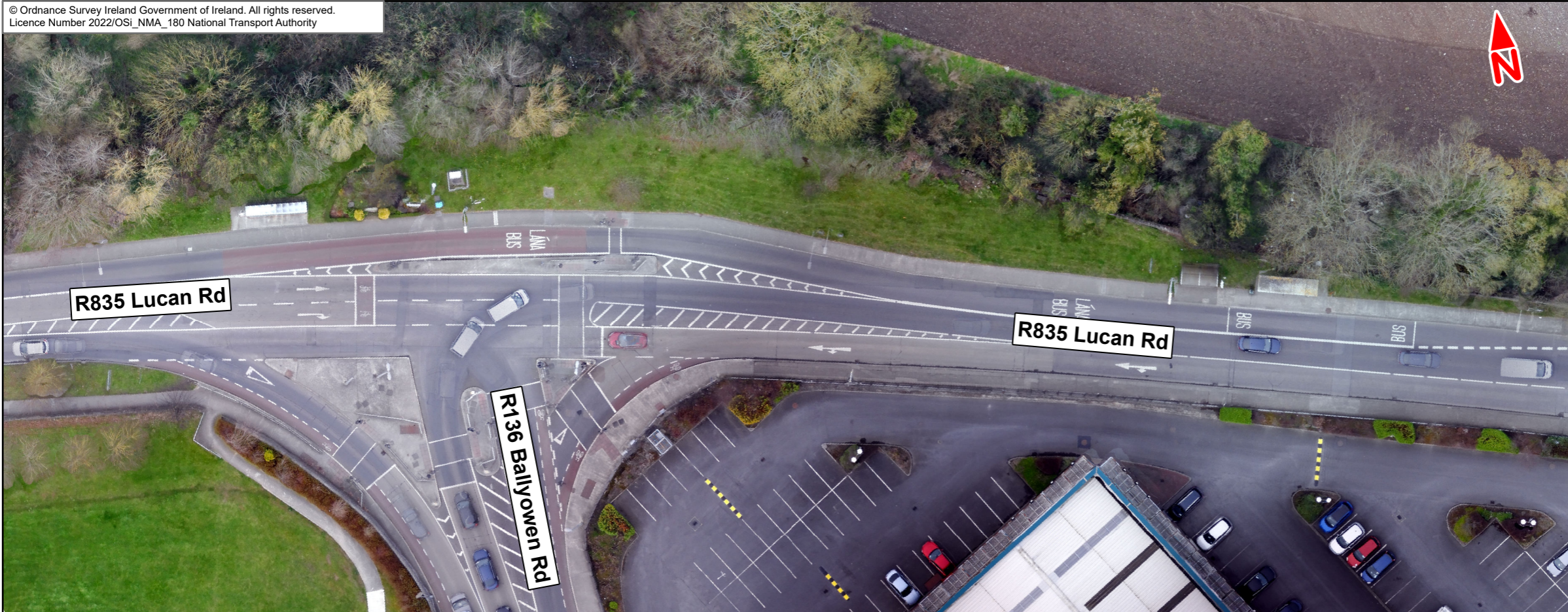
A) R136 BALLYOWEN ROAD/R835 LUCAN ROAD SIGNALISED JUNCTION
