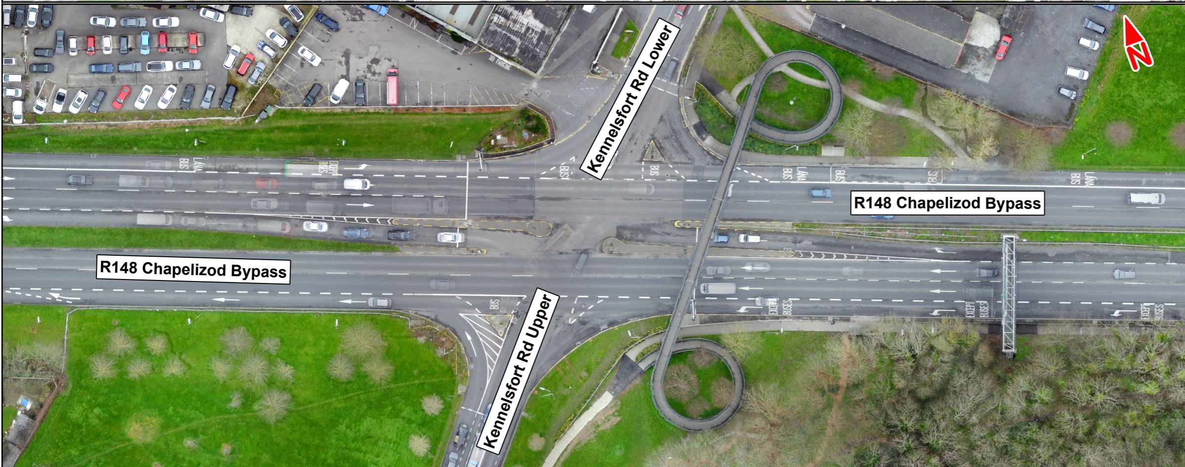
B) R148 CHAPELIZOD BYPASS/KENNELSFORT ROAD JUNCTION
