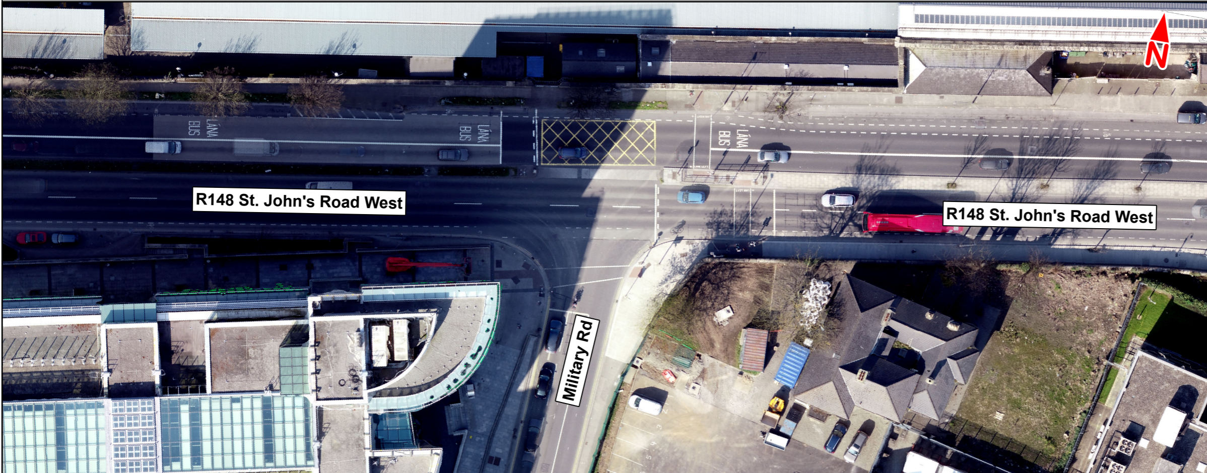
B) R148 ST. JOHN'S ROAD WEST/MILITARY ROAD JUNCTION
